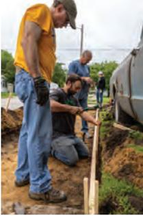
The sidewalk in Doug's front yard was deteriorating and he received a notice from the city. Volunteers were able to remove the old sidewalk and replace it with 27' of new sidewalk.
